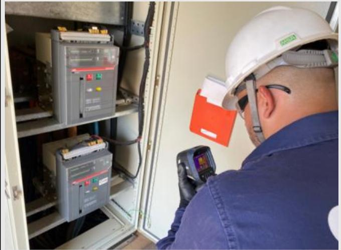
A technician wearing a white hard hat and safety glasses is using a thermal imaging camera to inspect electrical components inside an open metal cabinet. The components include two large grey units with red and green indicators. A red folder is attached to the technician's hard hat. |      |
